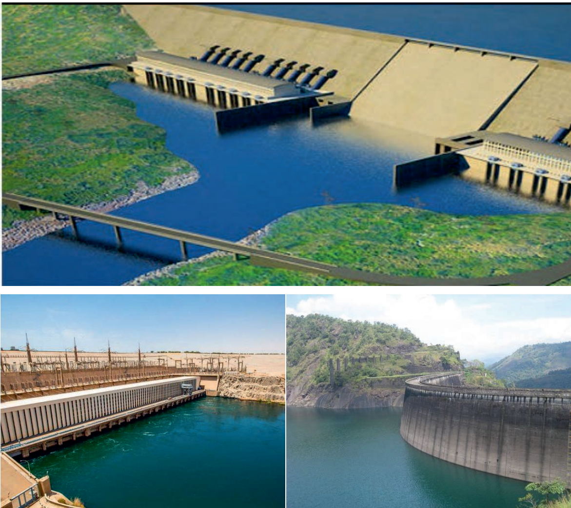
Figure 3.3: Dams on Trans-boundary Waters: GERD, Aswan and Sambangalou Top to down respectively.
