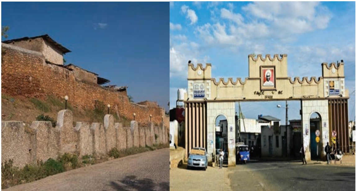
Figure 8.9 Harar wall (Jegol) and the main gate of Harar City (source: UNESCO site)
